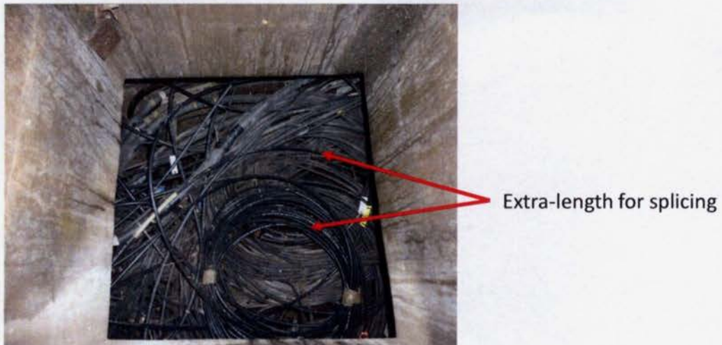
Figure 10 – Extra-length for splicing
